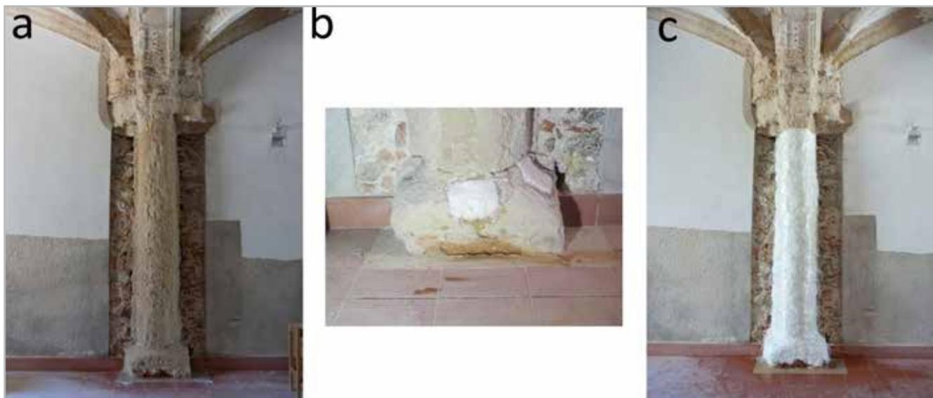
**Figure 3.-** Intervention of conservation; (a) removal of cement mortar, (b) the preliminary test of absorption with cellulose pulp ARBOCELL BC1000 and (c) the cellulose pulp applied over the entire surface of the column.
