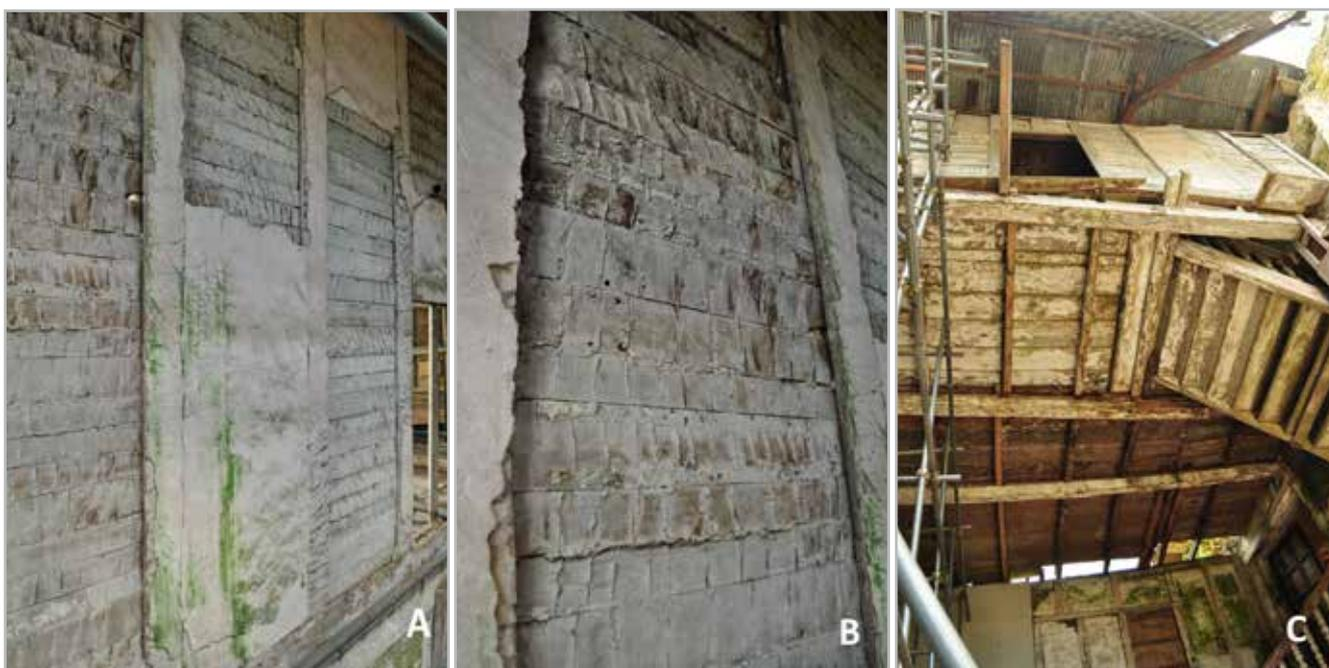
**Figure 2.-** Wall partition using the *tabique Pampango* (wattle-and-daub) technique. (A) and (B) shows the daub collection site with the exposed wattle frame. (C) is the view of the wall partition inside the 19<sup>th</sup> century Loboc church convent
