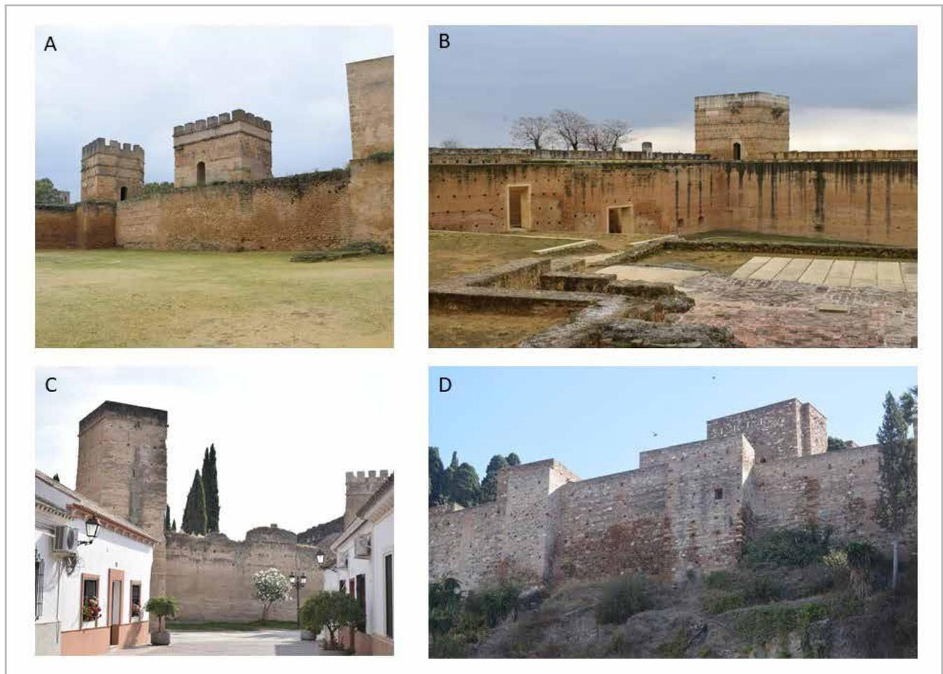
**Figure 1.** - A) Rammed earth lined with stone, Alcalá de Guadaira Castle (Seville); B) View of simple rammed earth, Alcalá de Guadaira Castle (Seville); C) View of simple rammed earth, Palmar del Río (Seville); D) Rammed earth lined with brick and stone, Alcazaba of Málaga.
