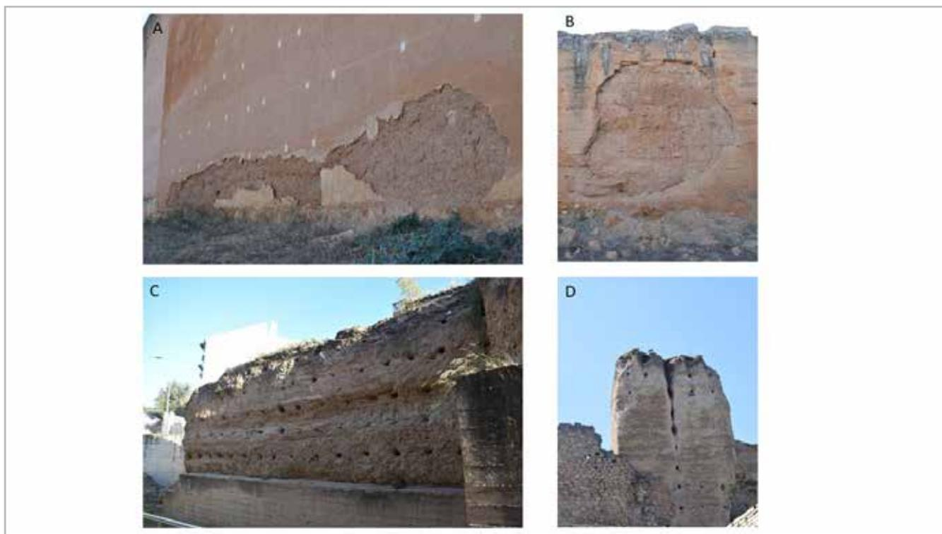
**Figure 2.-** A) and B) Displacements identified in the urban wall of Niebla; C) Erosion identified in the Alcazaba of Córdoba; D) erosion and fragmentation in the fortress of Marchena.
