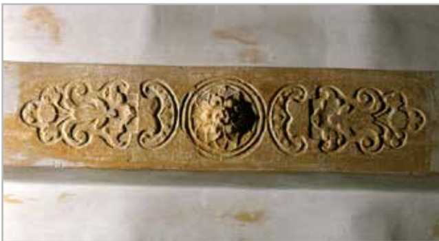
Figure 1.- Dordrecht Berckepoort. Renaissance clay plaster ceiling with stamped ornaments intaglio and casted lionheads and flowerbulbs, 1562. ©W. Freling.
