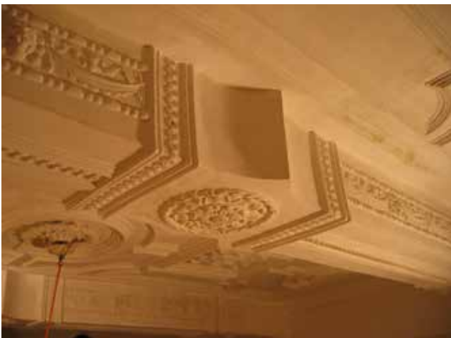
Figure 2.- Zutphen oude raadhuis. In the hall stuccoed nudo bars with casted rosettes and lionheads 1639 stuccoworker Jan Craekenborgh van Cleef. ©W. Freling.
