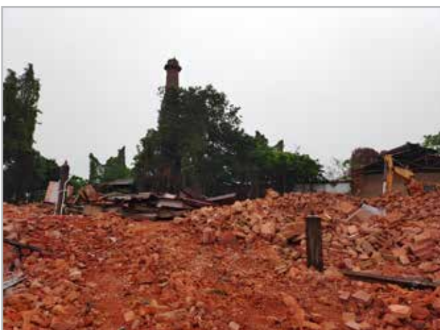
Figure 2.- Surviving Chimney of the now demolished Steam Loco Shed of the East Indian Railways at Allahabad (now Prayagraj). (Photo courtesy Vaibhav Maini)
