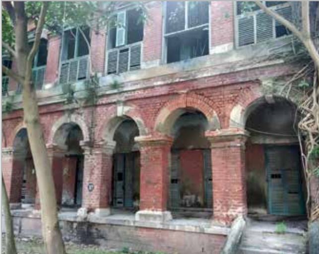
Figure 3.- Abandoned Salt Commissioner Office in Salt Golah, Howrah, West Bengal. (Photo by author 2016)
