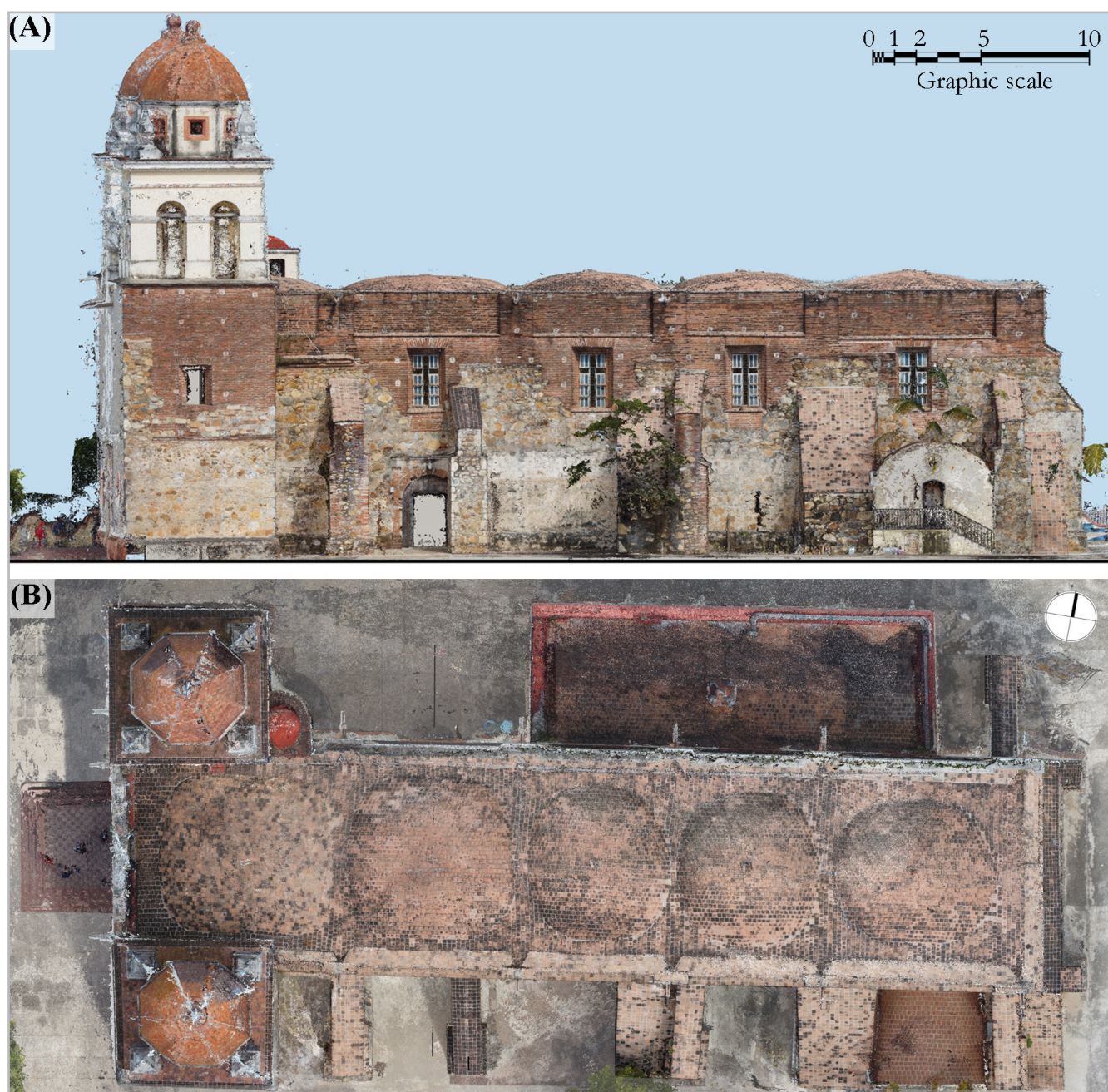
Figure 6.- Clean point cloud, within the SketchUp software, perpendicular views: (A) south elevation view and (B) rooftop plan.
