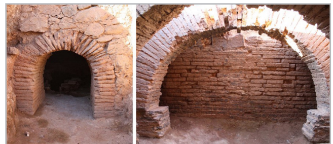
Figure 2.- A) Photo of the entrance to the bigger oven (H2) B) Photo of one semi-circular arch belonging to the H1 oven.
