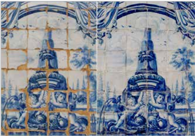
Figure 2.- Photograph of a detail of the panel before and after treatment with lime mortars and retouching with al fresco technique.
