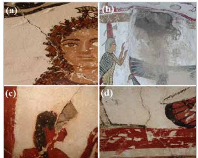
Figure 3.- Examples of deterioration forms on the wall decorations of El-Muzzawaka tombs (e.g. plaster loss and several cracks) (a), (b) the tomb of Petosiris, (c), (d): the tomb of Petubastis.
